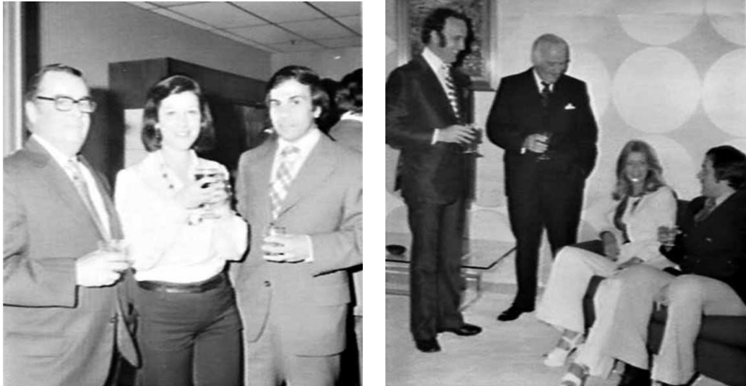
Figure 11 Photographs taken during Neata Fashions “Quest of Quest” entrants’ cocktail party held on 24 September 1973 give some indication of internal fit-outs within 119-127 Kippax Street at this time. Source: State Library of NSW.
