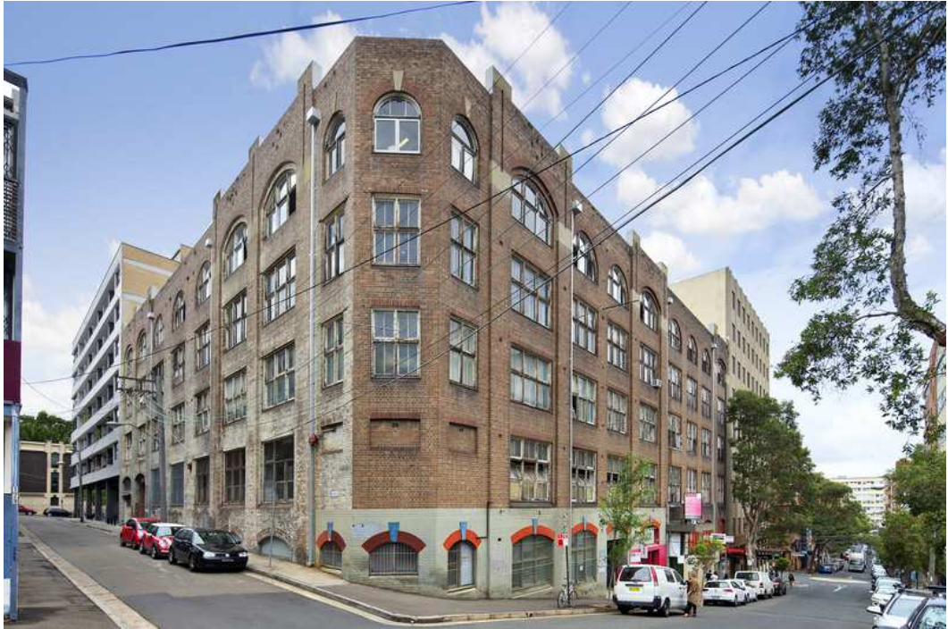
Figure 18 119-127 Kippax Street viewed from NE corner of Kippax and Lacey Streets.
