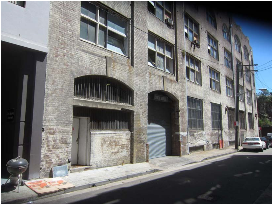
Figure 24 Fire egress and Loading Dock entry on Lacey Street
