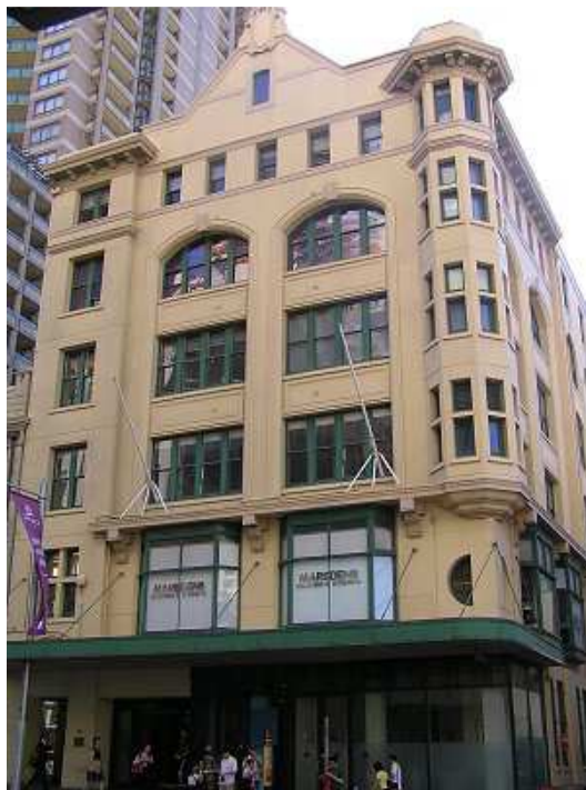
Figure 13 Metters Building. Source: State Heritage Register.
