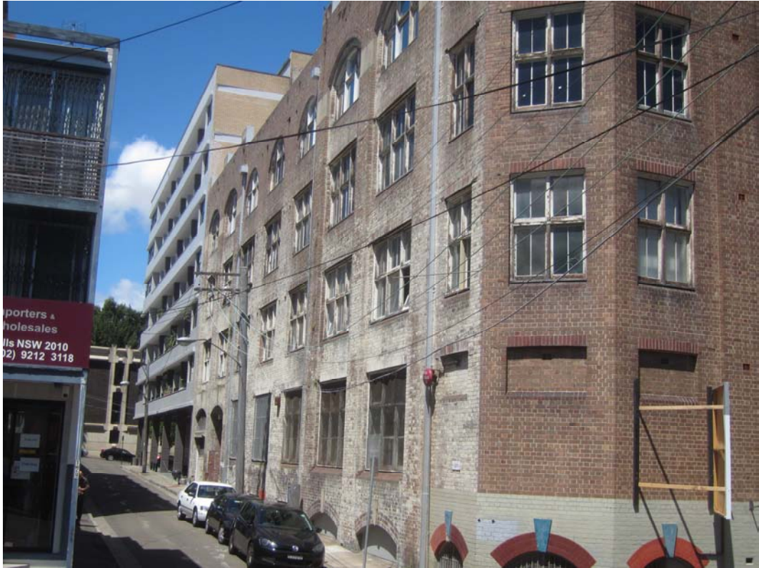
Figure 20 Lacey Street facade
