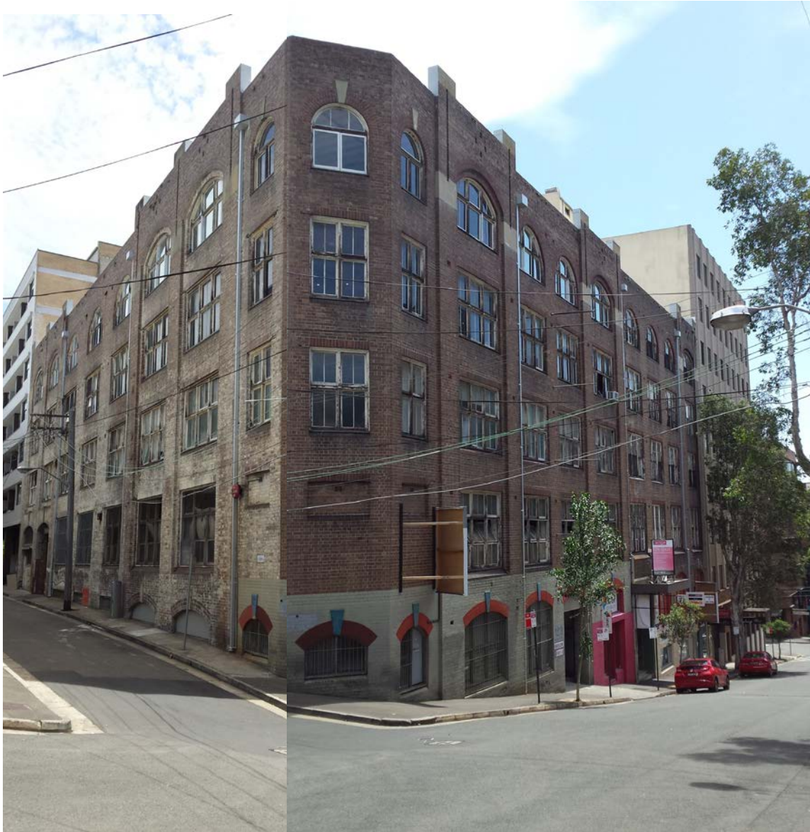
Figure 2: Photograph of Federation warehouse building at 119-127 Kippax Street, Surry Hills
