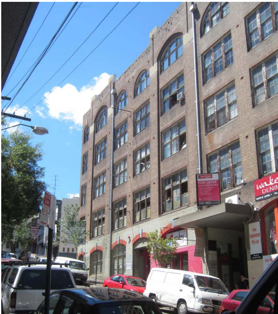
Figure 19 Kippax Street facade.
